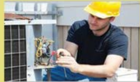
INSTALL AND REPAIR
