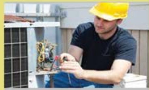
INSTALL AND REPAIR
