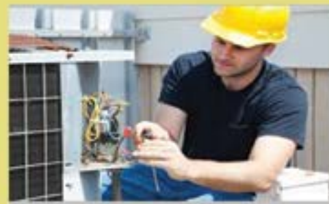
INSTALL AND REPAIR
