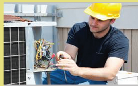
INSTALL AND REPAIR
